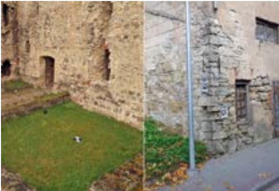
Survey markers when surveying buildings (author: M. Kaļinka)
