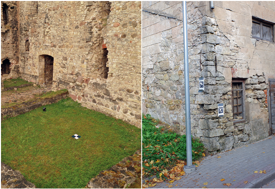
Survey markers when surveying buildings (author: M. Kaļinka)
