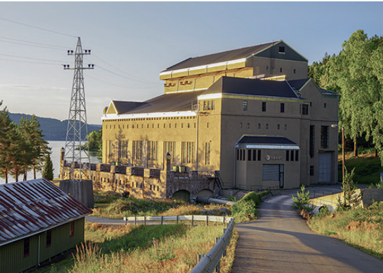
Hakavik power station. (author: Stig Storheil/NVE)
