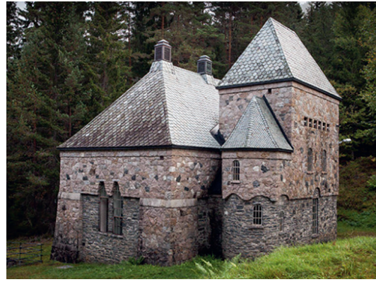
Longerak power station. (author: Stig Storheil/NVE)
